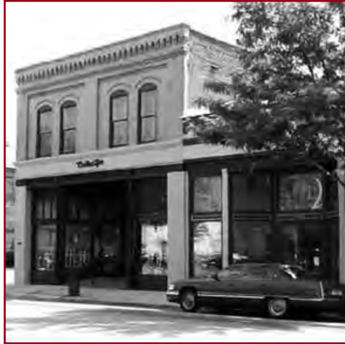
Bennettsville’s revitalization efforts have been successful in part because of the heavy investment in mixed-use renovations of historic buildings along Main Street.
